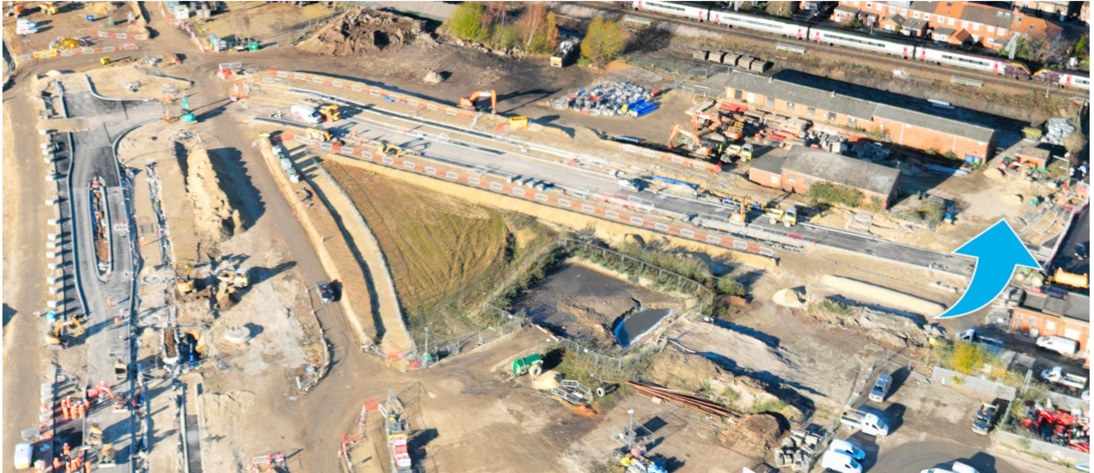
New link road showing connection into Leeman Road:
