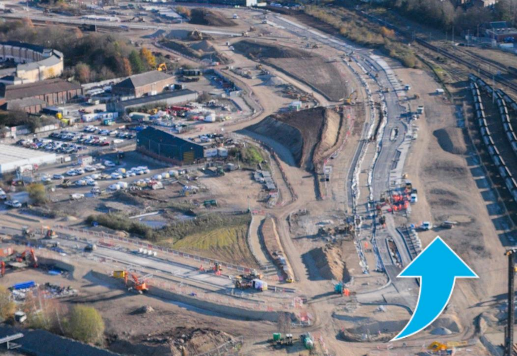
New link road showing blacktop and pavement installation
