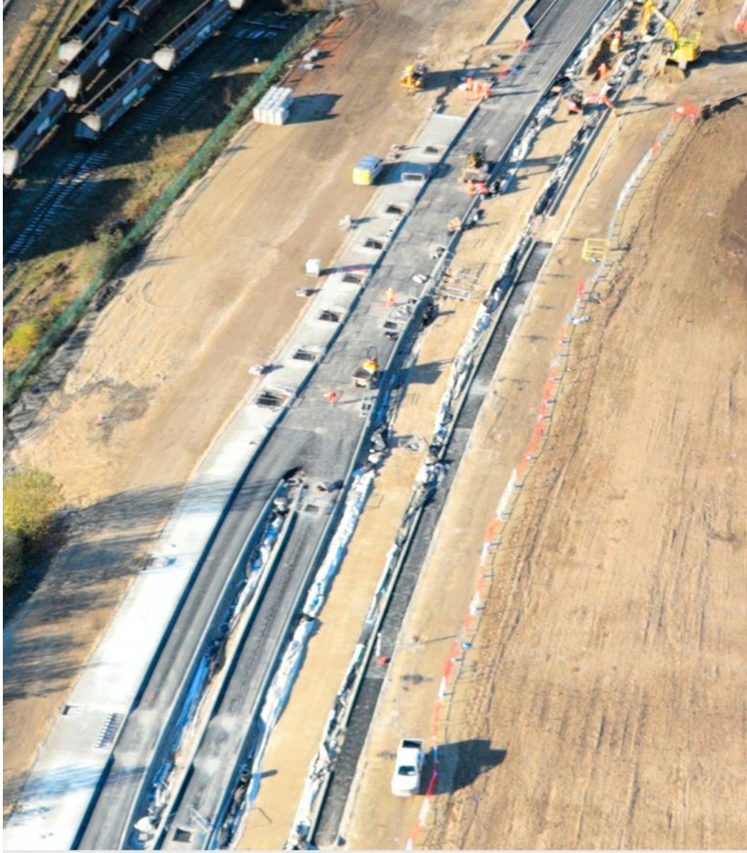
Part of the new link road showing blacktop, pavements and tree pits
